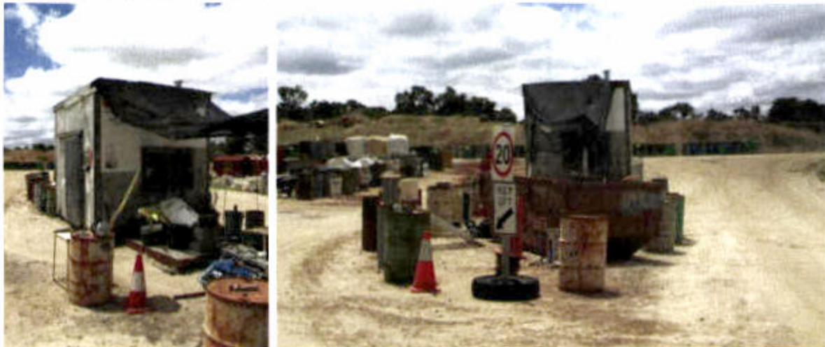
Figure 3-7. Existing gatehouse at the DWMF
