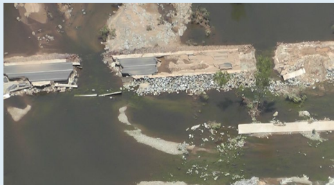
Hillside - Marble Bar Road (severe washout)
