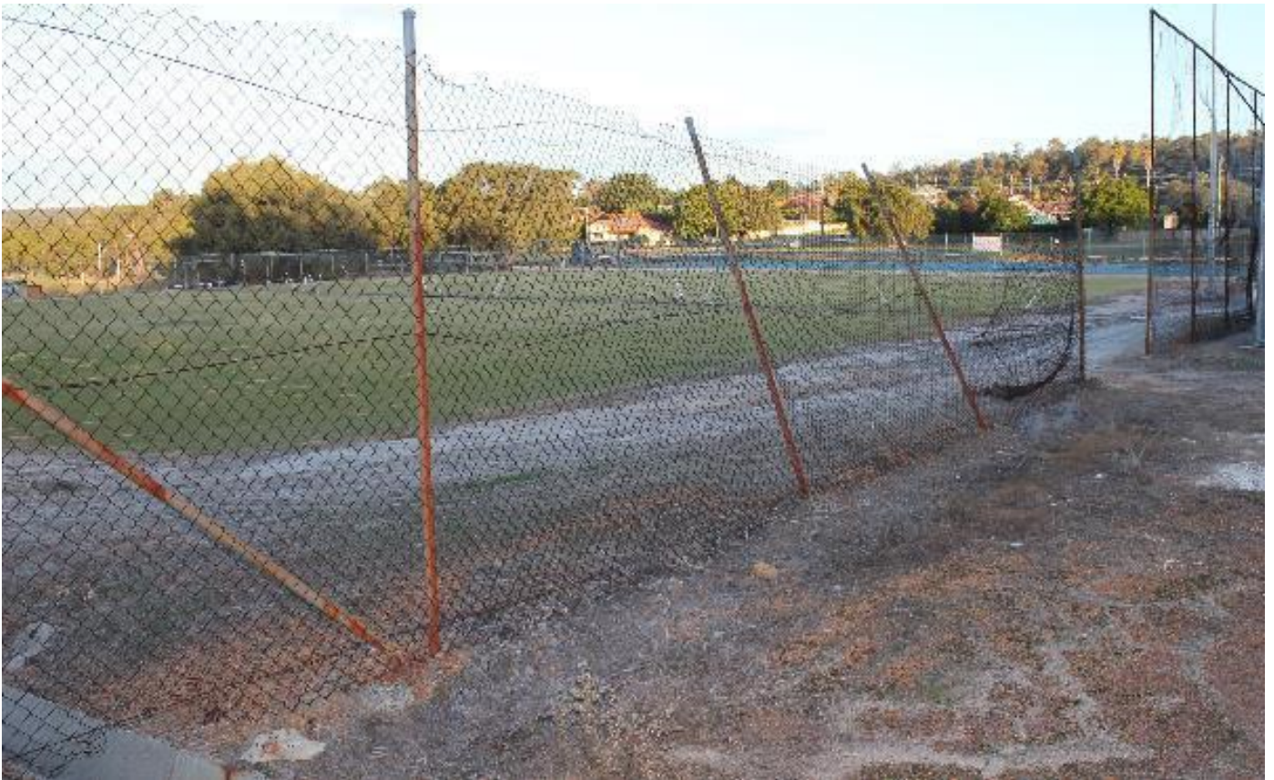
Figure 5 - Fencing in very poor condition and not functional
