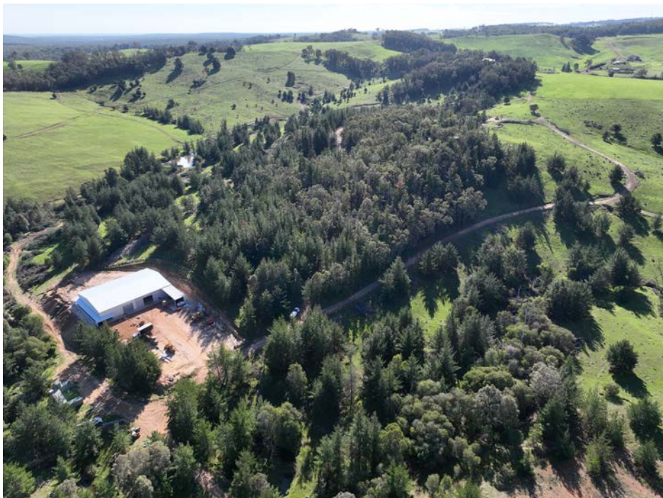
Figure 15 Processing shed in the south showing the tree protection
