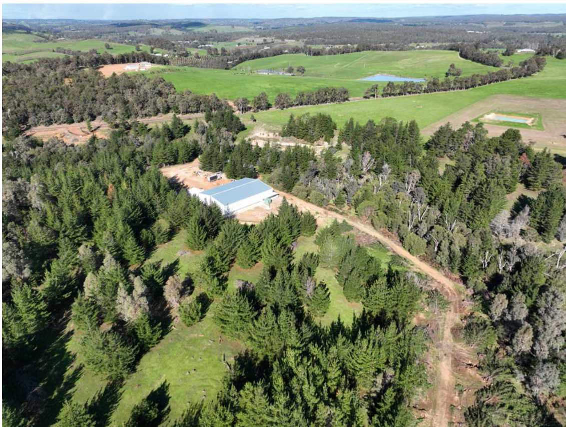
Figure 6 Overview of the new processing shed in the south
