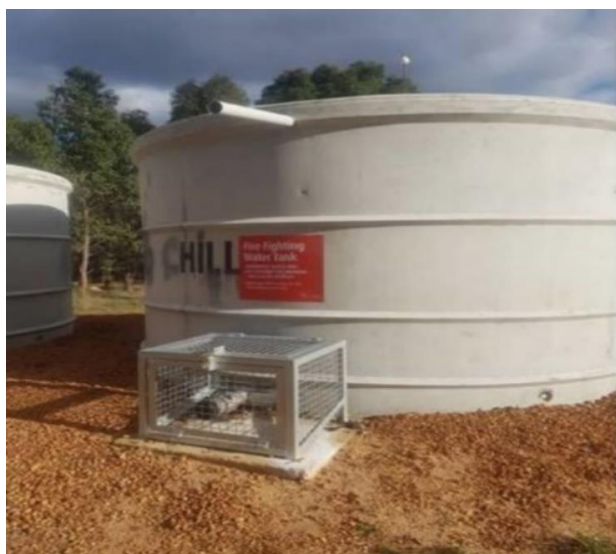
Strategic 47,000 Litre Concrete Tank & Protected Fittings
