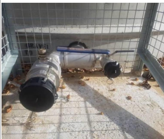
Strategic 47,000 Litre Concrete Tank & Protected Fittings
