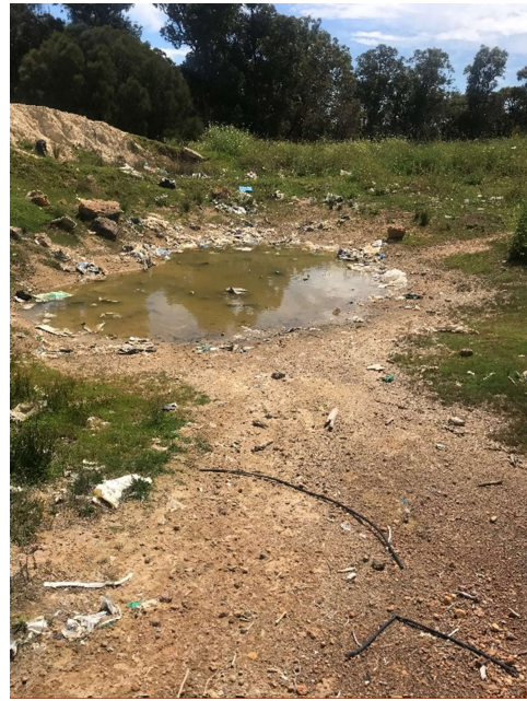
Photograph 14: Ponding stormwater at the northern corner of the landfill.
