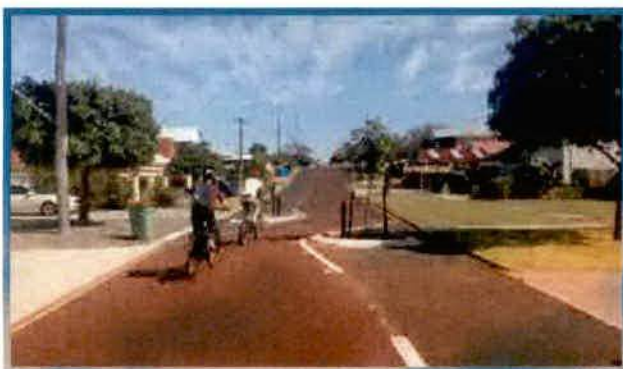
One-way slow point used for traffic calming and to switch formalised parking to other side of the road
