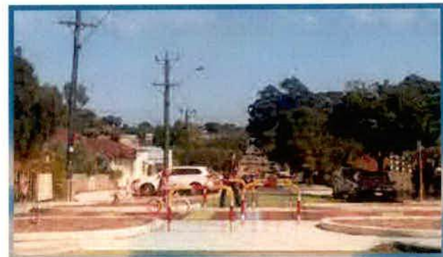
Mid-block road closure used to reduce traffic volumes
