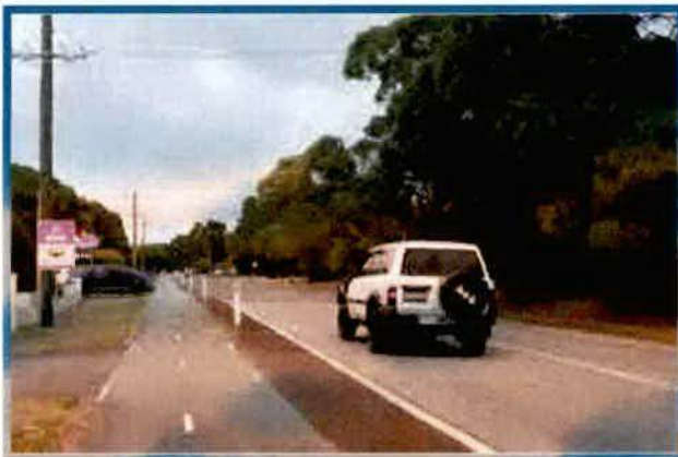
Bike lane separated with flexible plastic bollards
