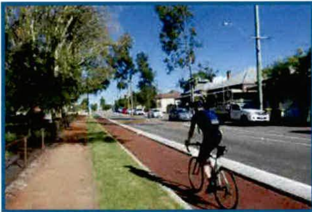
Bike lane protected with concrete kerb
