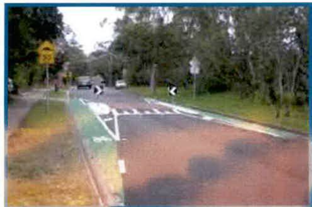
One-way slow point with bicycle-bypass facilities
