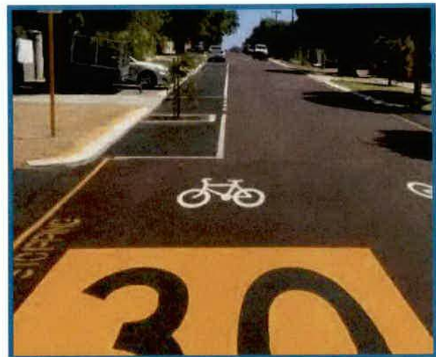
Road narrowing achieved through formalised car parking
