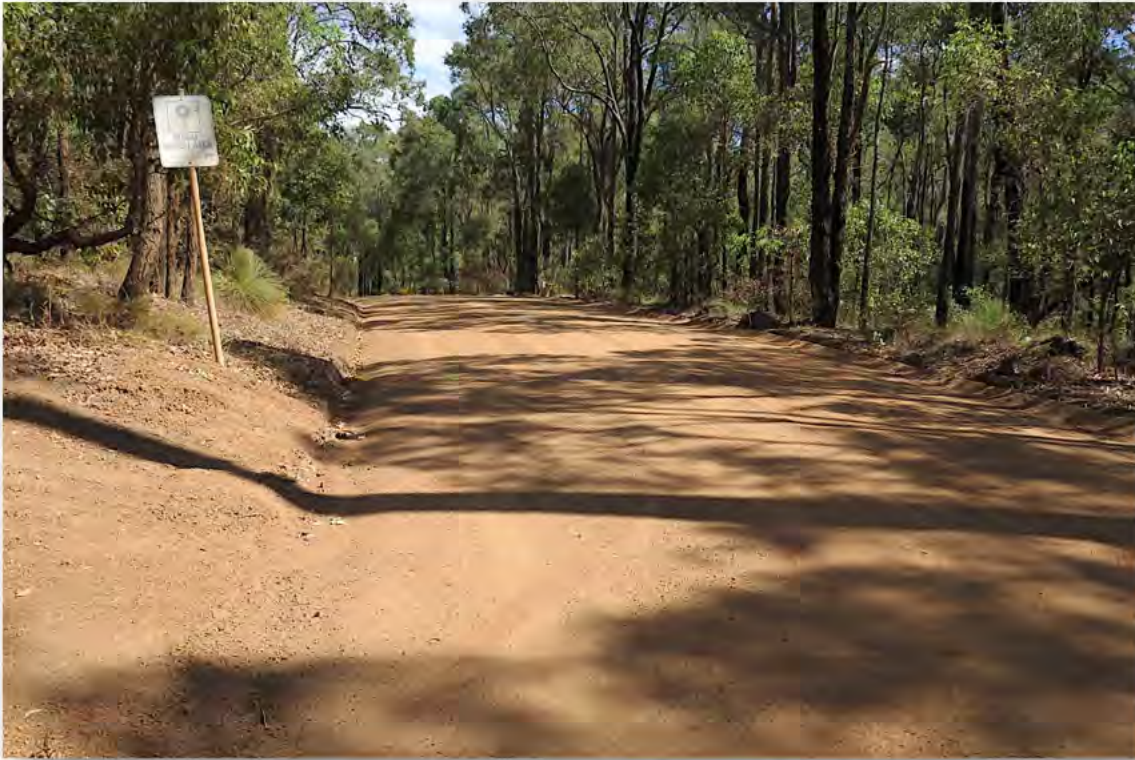
Figure 11: Spring Gully Road at entrance, view west
